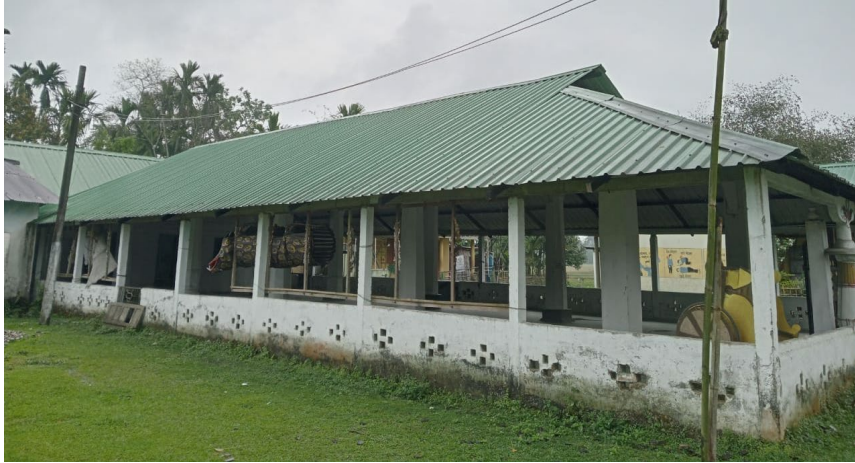
Figure 2.1: Typical Namghar Building
